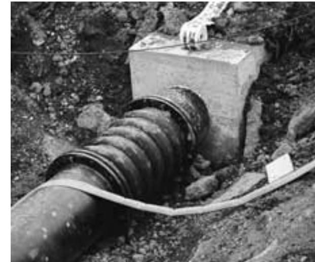
Beside a manhole
